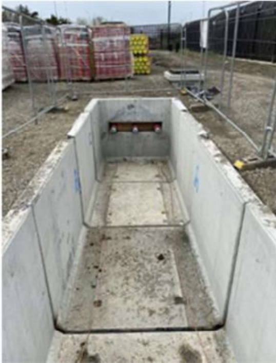
Figure 2-8: Typical Set-Up of HV Cable Pulling Procedure
